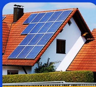
Solar Energy Storage
